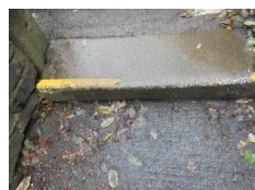
Nosing needs repairing
