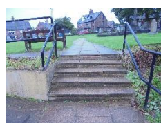
Nosing needs repairing
